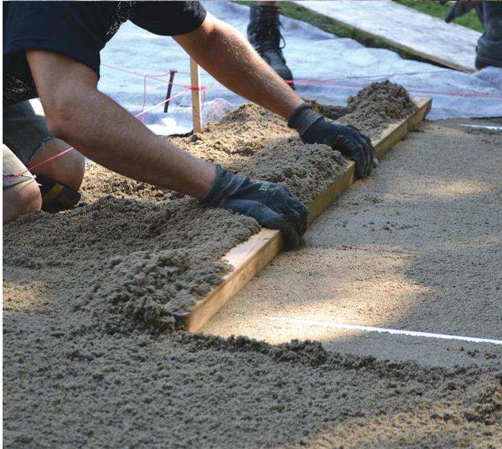
**STEP 3 • Addition of Geo-Fabric (non-woven Gator Fabric 4,4) levelling and compacting bedding sand**
