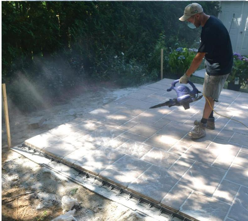
**STEP 6 • Sweeping and Compacting of the Gator Maxx G2 Polymeric Sand**
